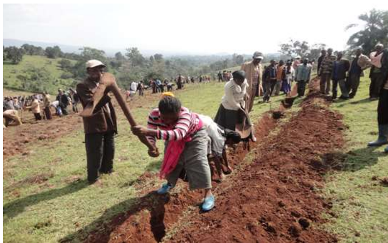
Figure 1. Soil and water conservation structure under construction. Source: Yericho Berhanu.
